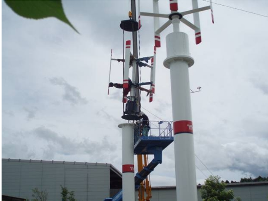
Fig.4.4 Building Vertical axis wind turbine
