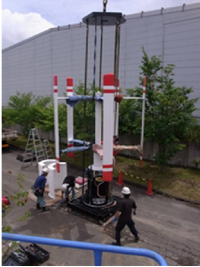
Fig.4.4 Building Vertical axis wind turbine
